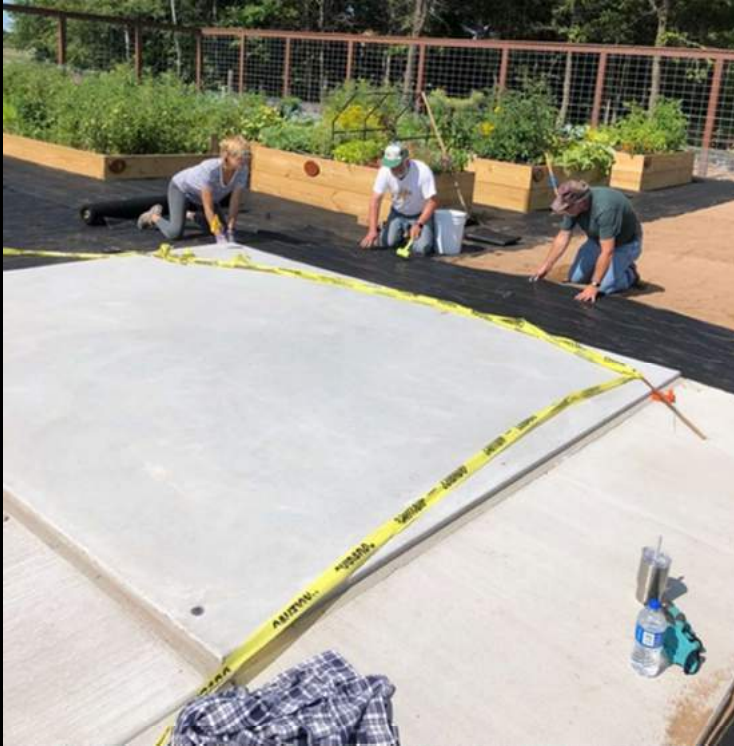
The garden shed slab is poured . . .
